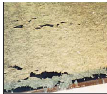
The floating sludge blanket-a mass of solids formed by the microbubbles that have captured and floated the pin floc to the surface-is easily removed with a mechanical skimmer or by hydraulic overflow
